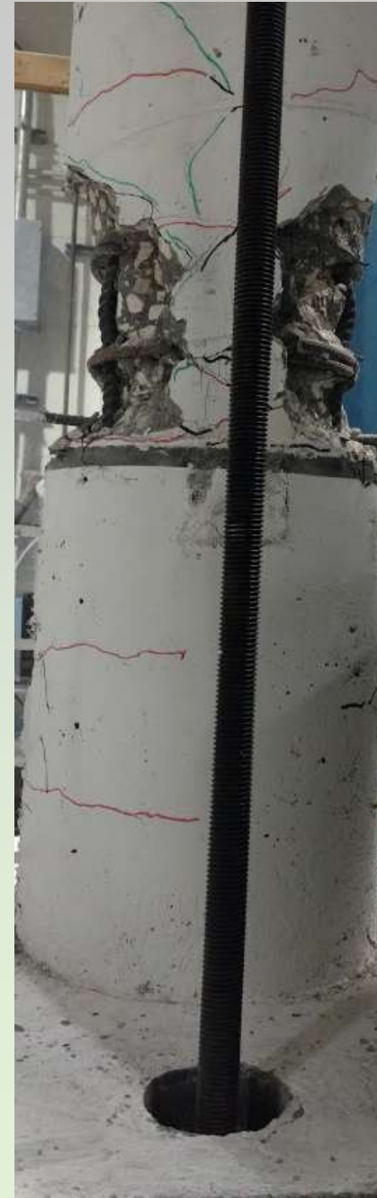
UNIT 11: Column & footing repair (UHPC 4% fiber) Symmetric repair
