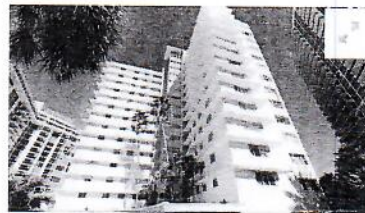
Carlton Terrace at 10245 Collins Ave., Bal Harbour.
