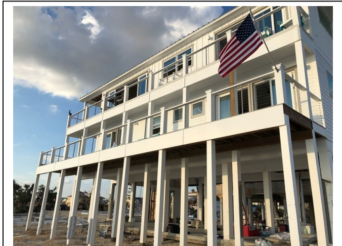
Figure 7. This home, built in 2017, is elevated higher than the minimum required by the FBC Residential and was designed for site-specific conditions. “Sand Palace,” concrete house in Mexico Beach after Hurricane Michael (Prevatt).
