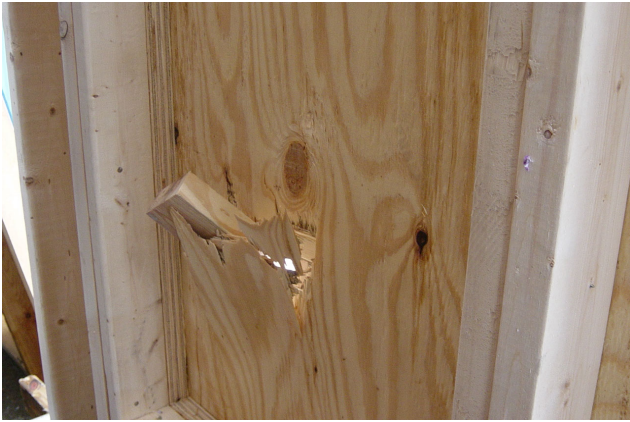
Figure 2-1. Typical 4.5 lb. 2x4 Missile Impact on Plywood Panel
