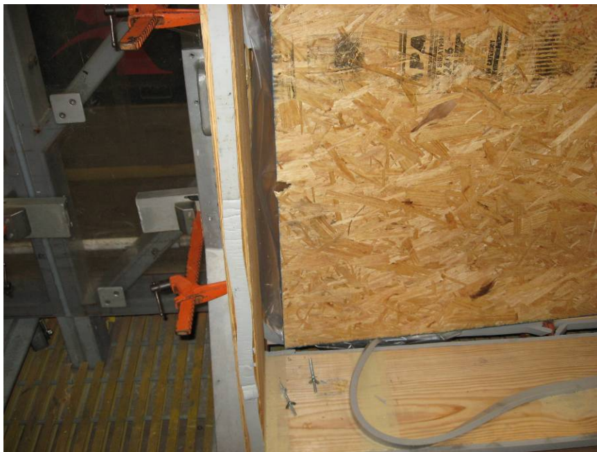
Photo No. 6 Specimen # 2 The two middle fasteners pulled through the plywood transferring point loads to the two end fasteners causing them to pull away from the 2x4 substrate and split the host wood bucking
