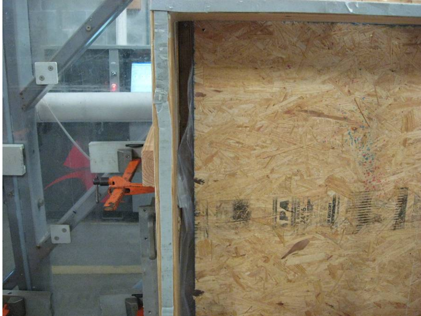
Photo No. 5 Specimen # 2 Failure on left side at 30.0psf
