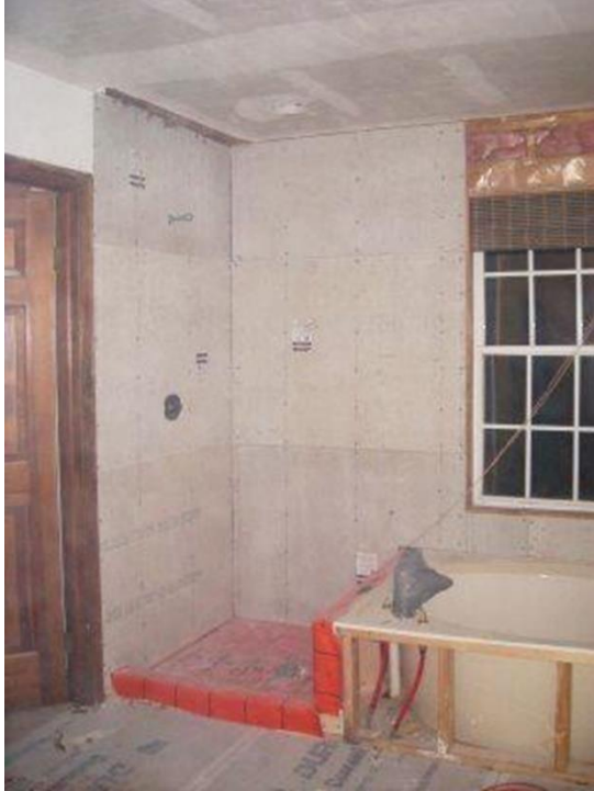
This is another picture of a shower liner and how you apply it.
