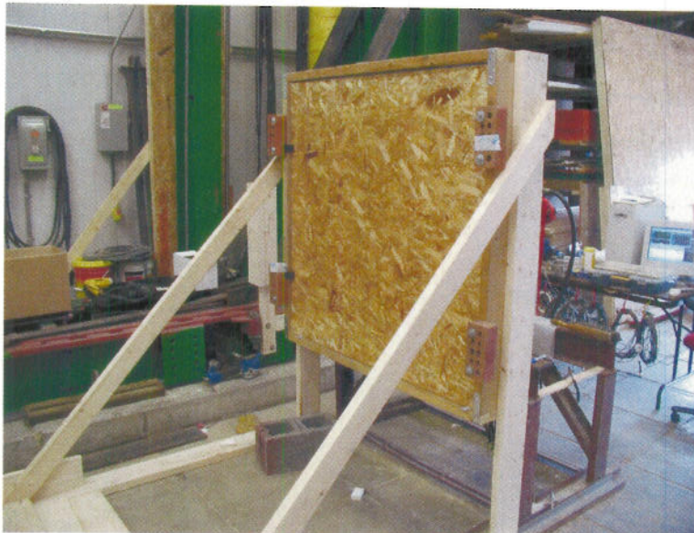
Figure 2. Test Frame with panel mounted to brick with Plylox™ clips.
