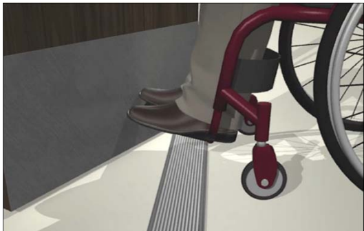
Kick plates can be used to protect door
