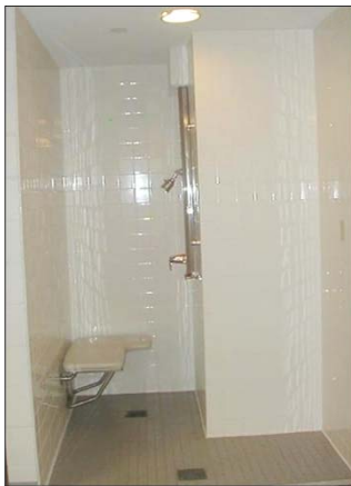
Common error: Insufficient space at seat wall
