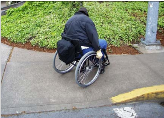
Lack of space at top makes curb ramps difficult to use
