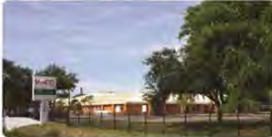
VizCO Corporate office in Bradenton, Florida.
