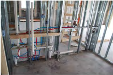
Examples of "mechanical walls" showing the abundance of utilities in this wall, demonstrating the need to provide more than 3.5"
