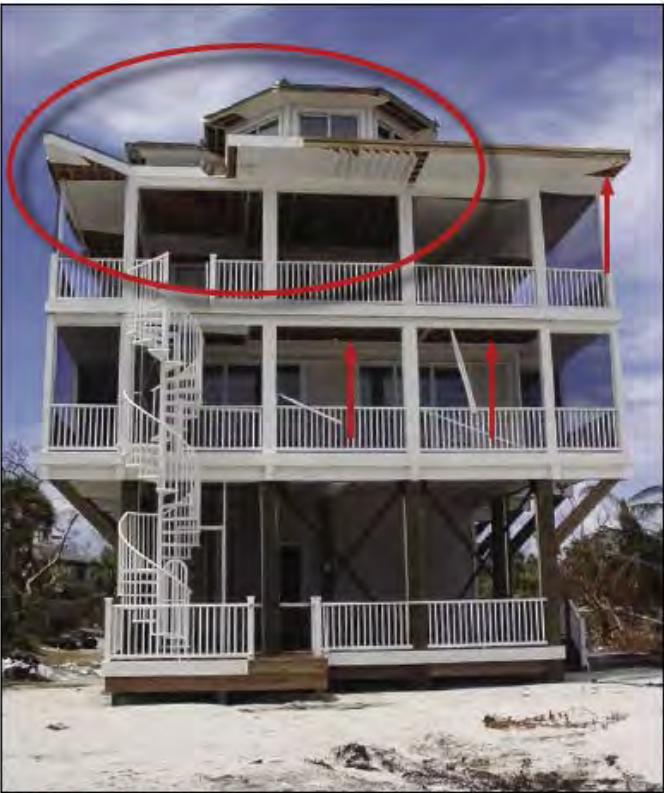
Figure 1. Missing soffit material.
