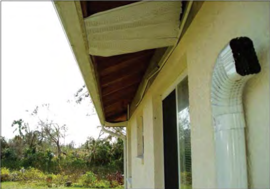
Figure 1. Missing soffit material.
