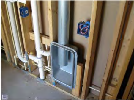
Examples of "mechanical walls" showing the abundance of utilities in this wall, demonstrating the need to provide more than 3.5"
