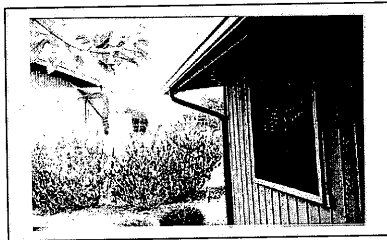
Figure 8.9 Existing Gutter and Drain Spout
