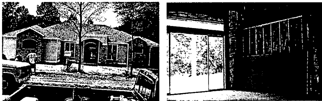
Figure 4.1 Jockey Club house under construction.
