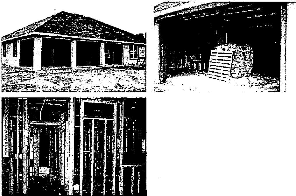
Figure 4.4 Parker Place house under construction.
