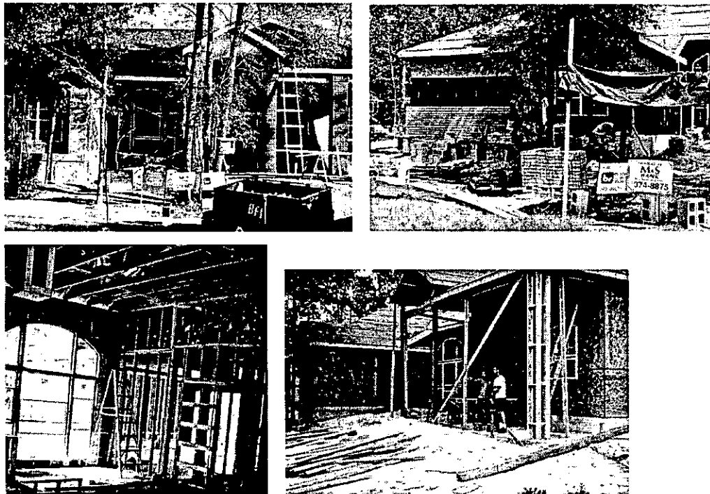
Figure 4.3 Haile Plantation house under construction
