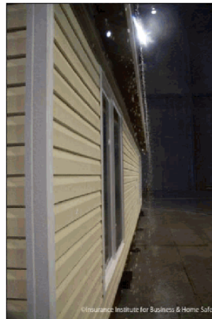
Figure 7 - Photographs of the water entry quantification testing for the open soffit case with the wall facing the wind flow: top) whole duplex; and bottom) close-up of the open soffit area.
