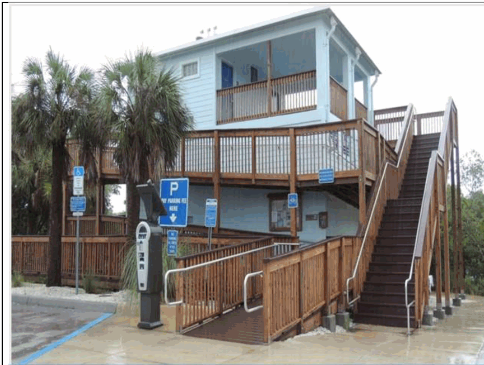
Figure 1. Florida, flood Zone V. Ramp wraps around entire building. Has composting toilets, battery and solar electric system, emergency plan requires pumping out tank and filling with clean water.
