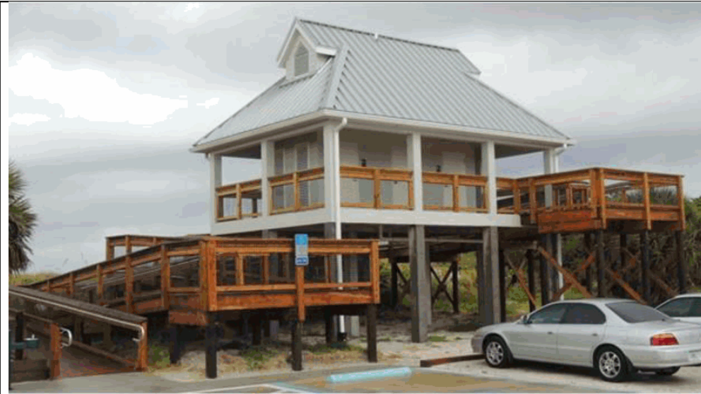
Figure 4. Southwest Florida, flood Zone V. Extensive ramp wraps around three sides.
