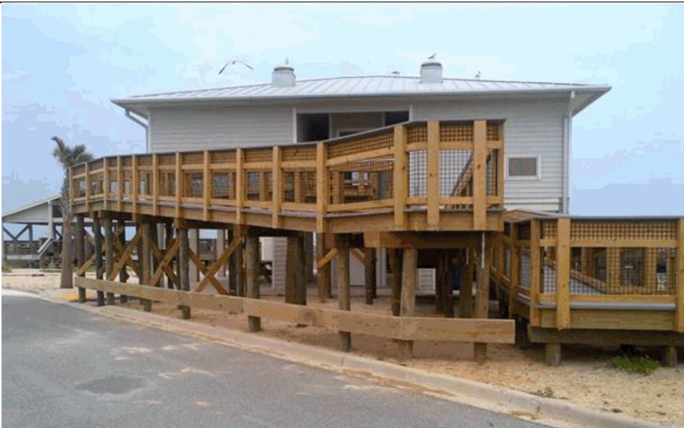
Figure 3. Florida, Gulf Coast, flood Zone V. Ramp built after original elevator determined to be unsustainable due to significant maintenance problems.
