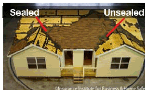
Figure 9 - Photograph of the front of the duplex after shingle and underlayment removal using high winds, illustrating the sealed roof deck (on the left) and the un-sealed roof deck (on the right).
