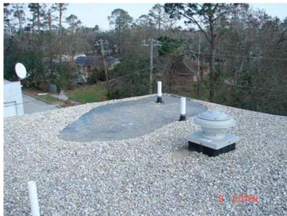
FIG. 5—Wind vortex formation on gravel roofs due to low parapet.
