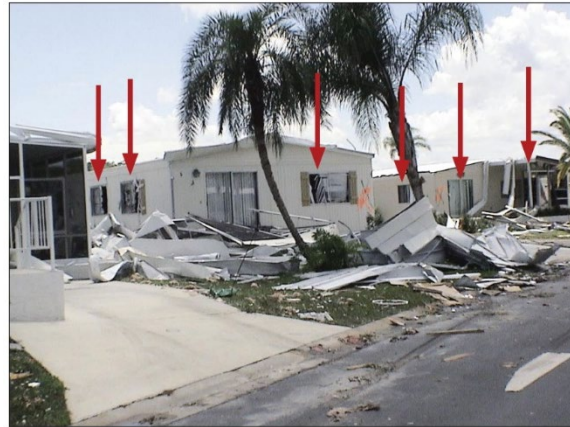
Figure 11. Wind-borne debris damage on windows caused metal roof panel and siding in Port Charlotte during Hurricane Charley (2004).
