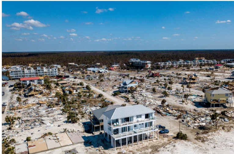
Figure 34. Widespread devastation to wood-framed single and multi-family residences in Mexico Beach with few survivors in areas with highest inundations (Source: New York Times)
