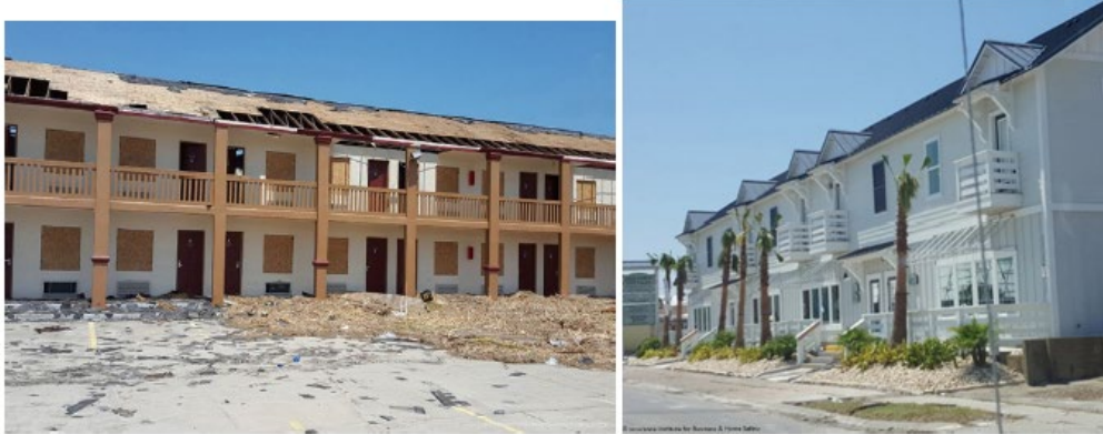
Figure 25. Comparison of two commercial buildings located 1 mile apart that experienced similar wind speeds during hurricane Harvey (2017) but performed very differently in Port Aransas North. The older construction was built in 1984(left) and newer construction was built in 2017 (right).
