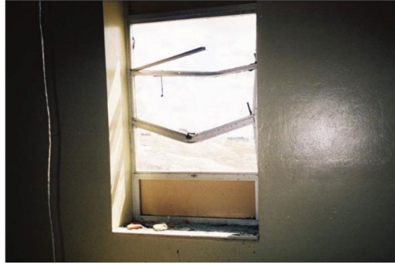
Figure 21. Broken window caused by wind-borne debris in a high school in Punta Gorda during Hurricane Charley (2004).
