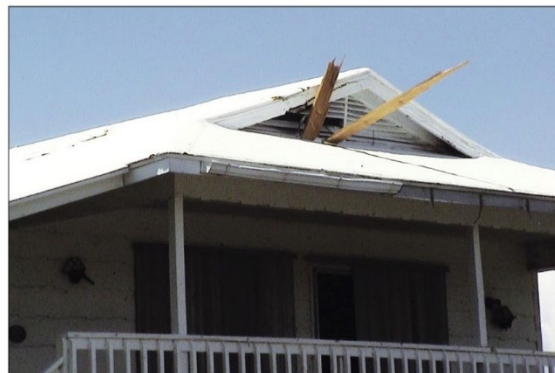
Figure 10. Impact of structural wood in the gable end in Pine Island during Hurricane Charley (2004)
