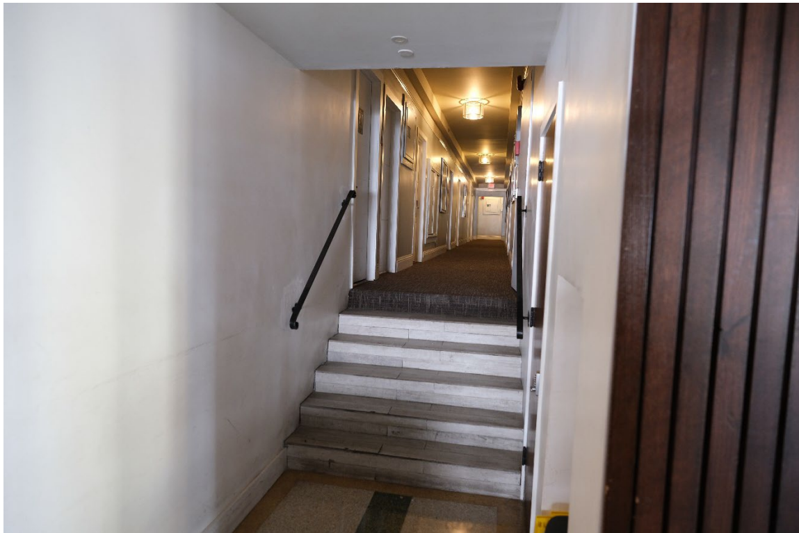
Stair from Lobby Level to First Floor
