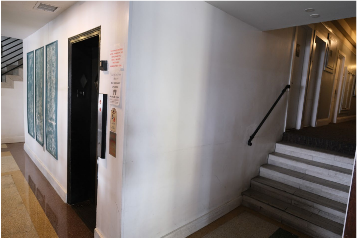
View showing Elevator, shaft side wall and stair to First Floor
