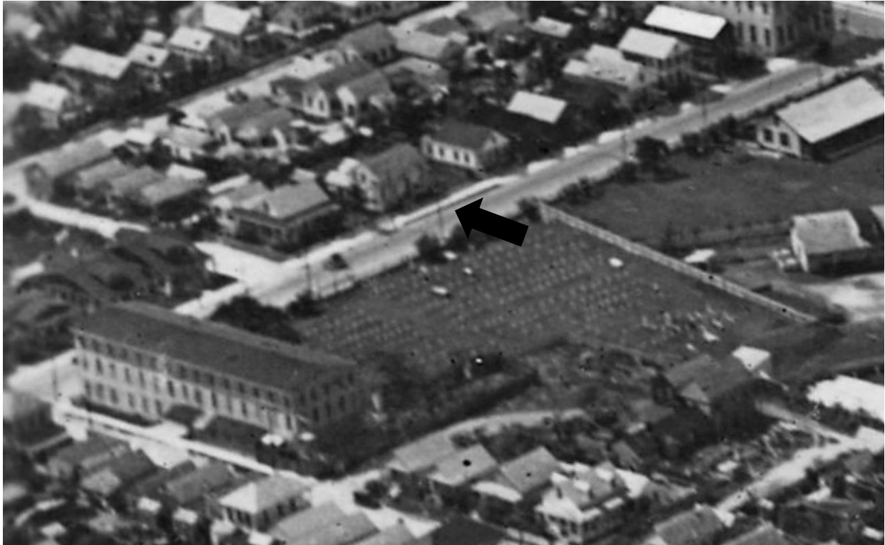
Circa 1920 aerial photo showing 624 White Street. (Key West Public Libraries via Flickr)
