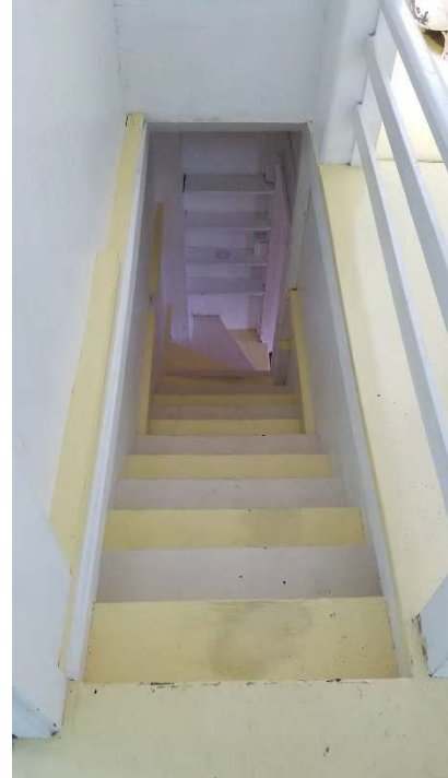
The interior stair, viewed from the second floor landing. The painted wood stair is very significant and probably original to construction.
