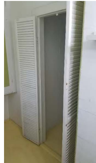
The louvered door leading to the second floor bathroom. This door is contemporary.
