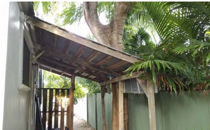
The side porch at the south side of the house covers a utility area used for a laundry, outdoor shower, a stone laundry sink and storage.
