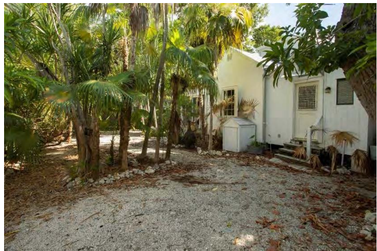
General view of the rear yard of 624 White Street.
