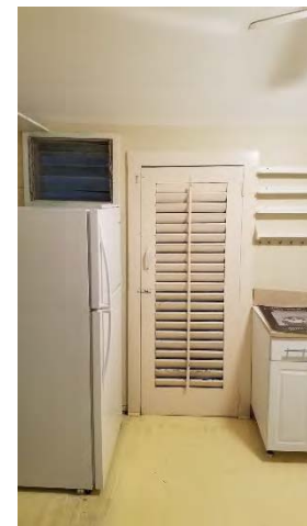
The painted wood louvered west door of the kitchen. This door leads to the west porch.
