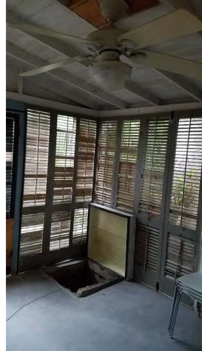
General view of the covered porch at the NW corner of the house. The porch is built atop the concrete cistern cover.
