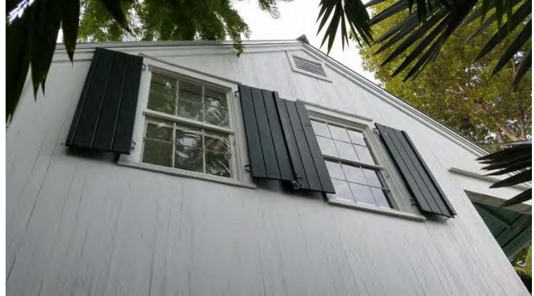
This view of the south façade of the house shows the painted wood vertical siding.
