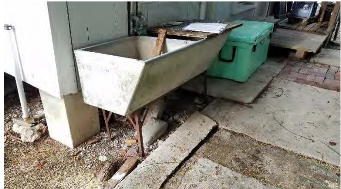
The cast stone laundry sink at the south side of the house. This sink probably dates to the early 20 th century.
