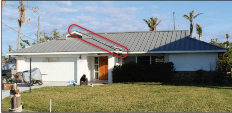
Figure 4-25: Typical hip cover damage on a metal panel roof (EWS: 115 mph; DWS: 161 mph) (St. James City)
