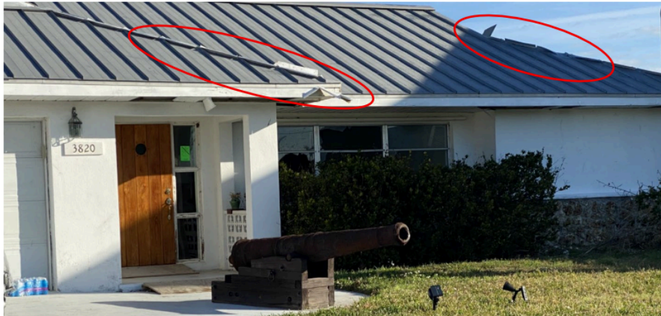
Figure 4-25: Typical hip cover damage on a metal panel roof (EWS: 115 mph; DWS: 161 mph) (St. James City)
