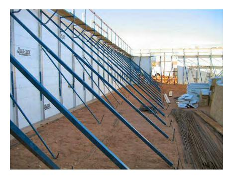
Figure 109: Bracing Tall Walls
