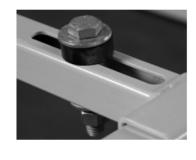
7. Mount unit to stand and insert in slot one 3/8"-16 x 1 ½" bolt, two 3/8" galvanized washers, one rubber washer, one 3/8" split washer and one 3/8" nut.
