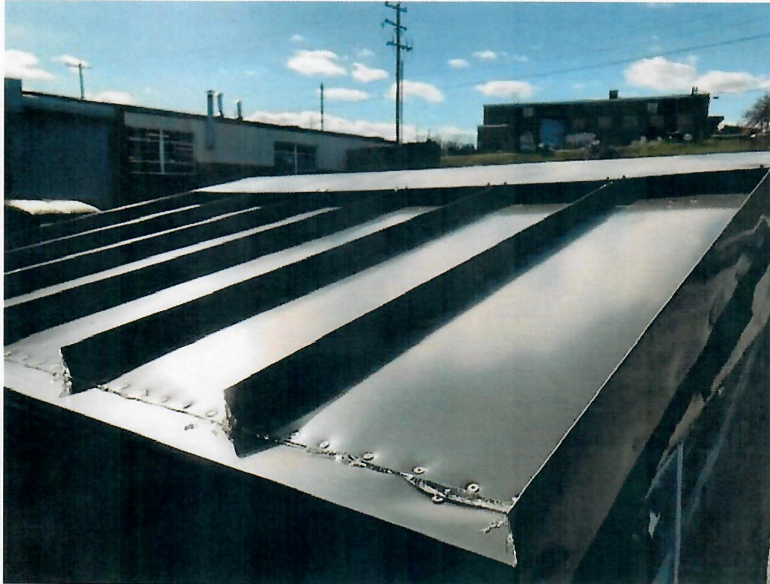
Photo No. 1 Top Side Before Testing
