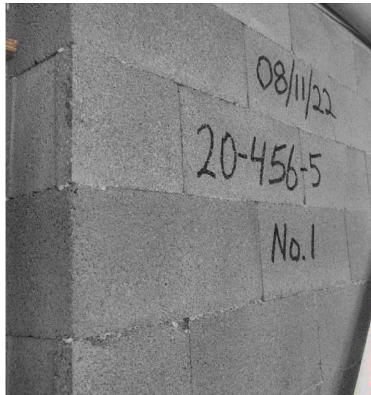
2 01 SAMPLE SYSTEM: CMU WALL WITH FBR ADHESIVE NOT TO SCALE ISOMETRIC VIEW
