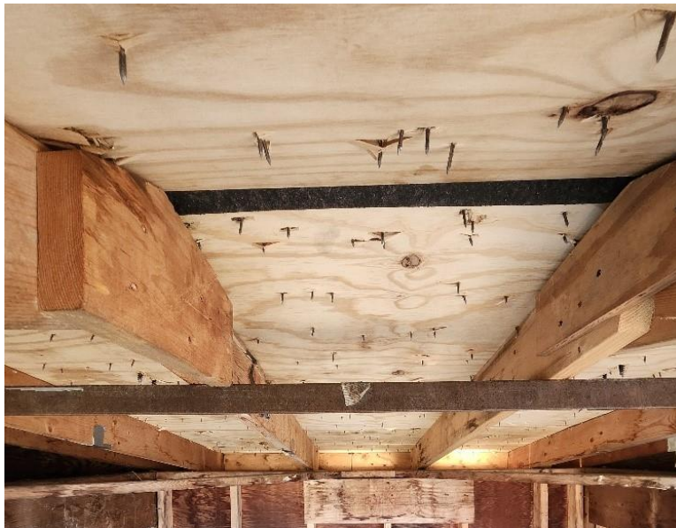
Photo No. 2 Underside Before Testing
