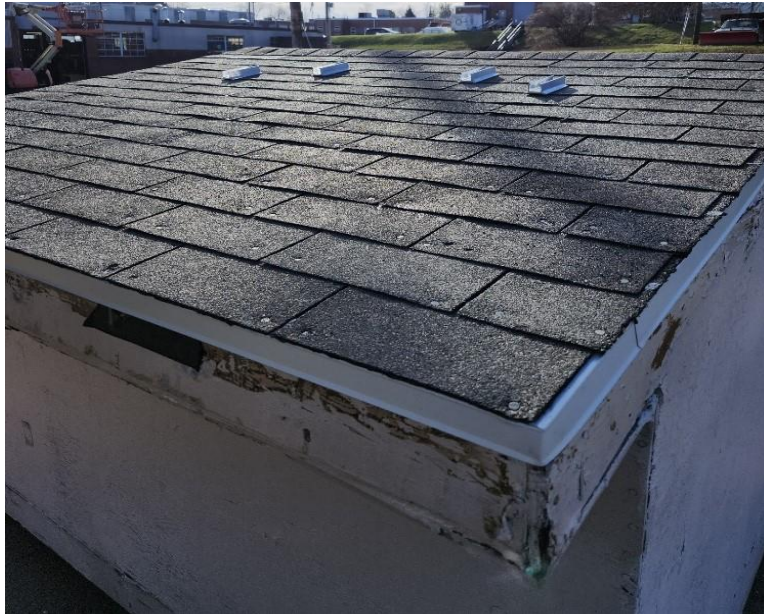
Photo No. 1 Top Side Before Testing
